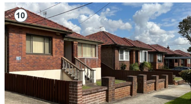
Single (1) storey brick dwellings situated along Kings Road which are elevated above street level with a small set of stairs, and low brick fence at the street frontage.
