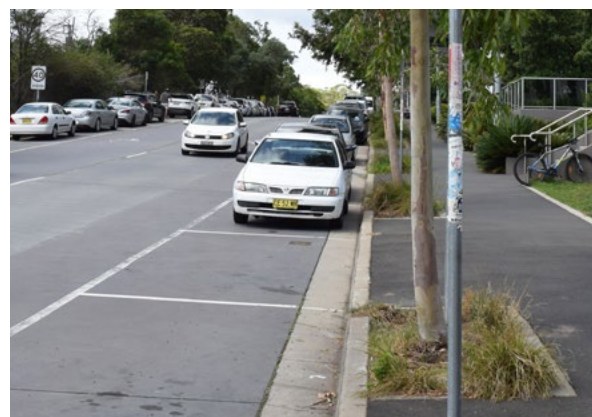
Parking spaces are to be marked to more clearly delineate their extents and to help prioritise street functions such as emergency access.
