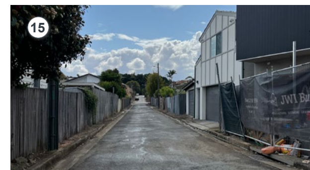
View looking north along Barnstaple Lane (rear lane). The rear lane redirects private driveway access away from the primary street frontage (Trevanion Street).
