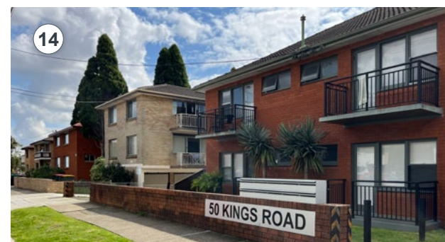
Two (2) to three (3) storey walk-up apartment buildings on the northern side of Kings Road.
