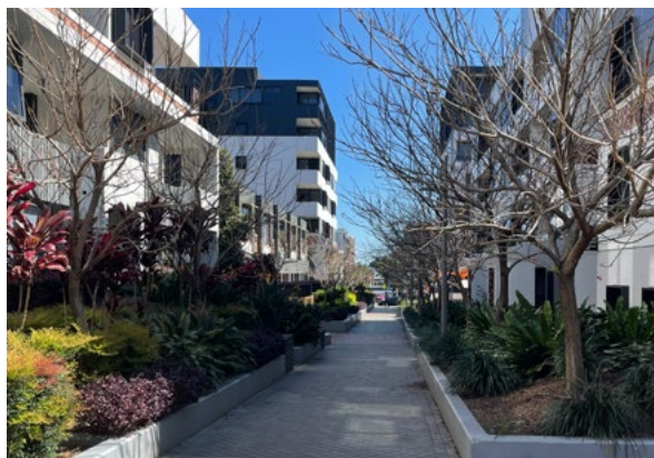
Buildings designed to face well landscaped and well designed accessible pedestrian links
